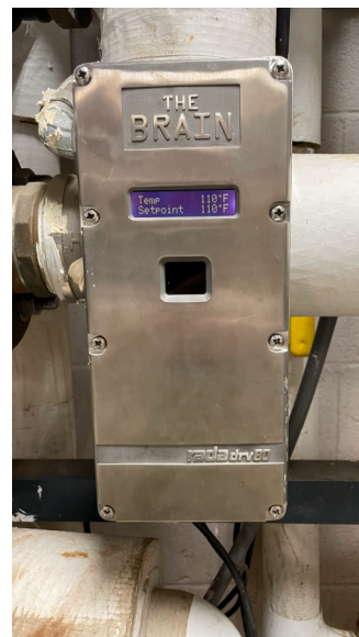
Figure 18: Thermostatic Mixing Valve
